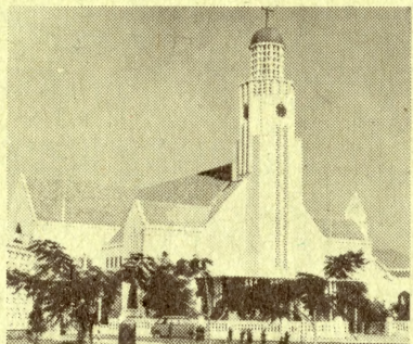
PROTESTANT CHURCH ... in Oranjestad. One of the town's finest landmarks is this modern new church. Although the church is painted gray, the quaint old houses sport the brightest paint jobs ... raspberry red, Delft blue, sunshine yellow and all other brilliant colors giving Oranjestad a charming kaleidoscopic effect.
